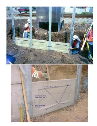
5. After installation of the lower panels and panels are secured in place with the brackets, the next panel is installed on top of the lower panel and secured in place with brackets. Refer to Detail Sheets 1 & 2 for specific brackets and assembly detail.
