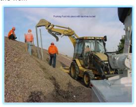
3. Position the first concrete panel into place to determine placement of the next post. Install the post in the proper location.
